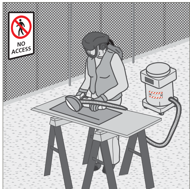
Figure 5: Controlled exclusion zone with restricted access
