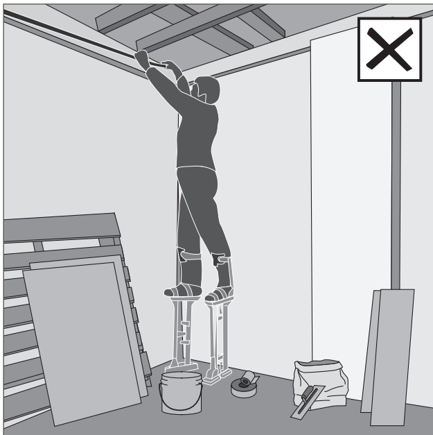
Figure 26 Inappropriate environment for working on stilts – poor housekeeping of floor surfaces.
