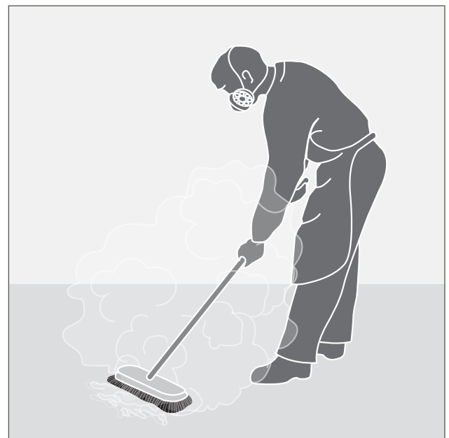
Figure 9(a): Before – Dry sweeping can create airborne lead dusts in the breathing zone
